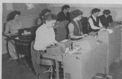
THE STORY IS TOLD on a card. These key punch operators have the task of operating the machine which puts the holes in detail cards. Skill and speed are necessary here.
